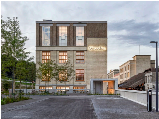
( https://divisare-res.cloudinary.com/images/c_limit,f_auto,h_2000,q_auto,w_3000/v1583763795/p_niklaus-fausch-partners-ag-johannes-marburg-givaudan-office-building.jpg ) © JOHANNES MARBURG
